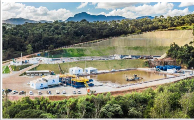
Conclusion of the Ferro-Carvão Stream Water Treatment Station
