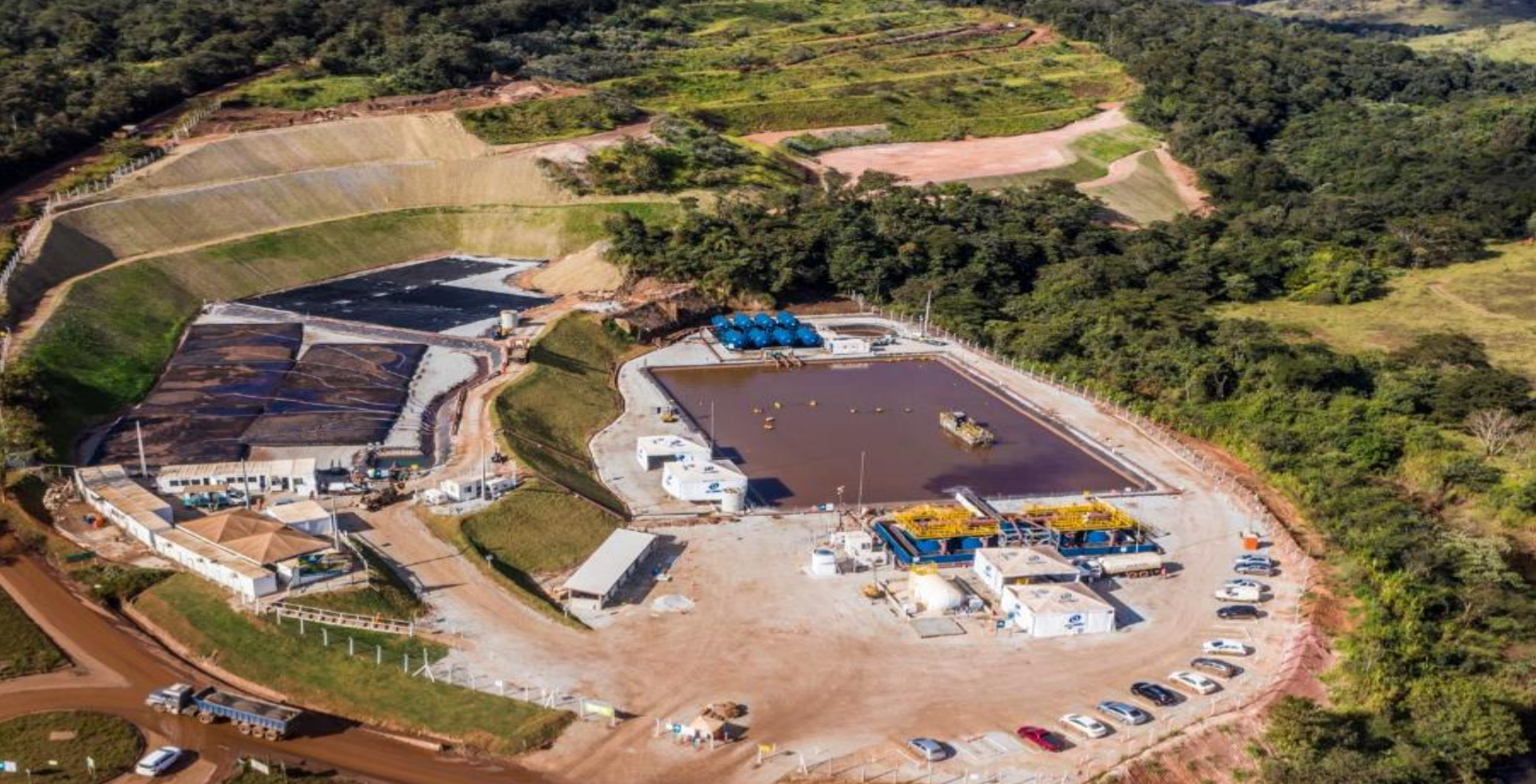
Conclusion of the Ferro-Carvão Stream Water Treatment Station in Brumadinho, MG
