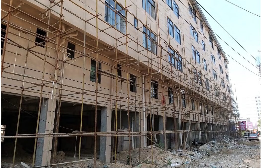
Another construction site in Otres Village, Sihanoukville. PC: Ivan Franceschini.
