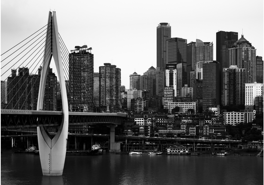
Chongqing, Dongshuimen Bridge. PC: Ivan G Shevchenko.
