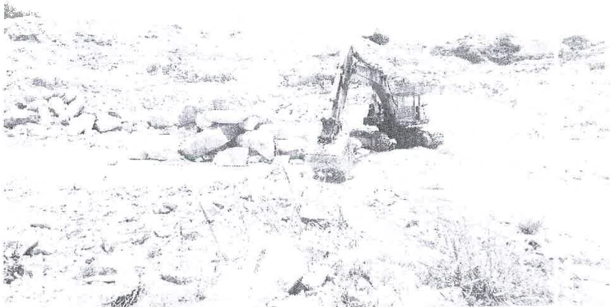
The current state of the blasting region with in the stone quarry project area
