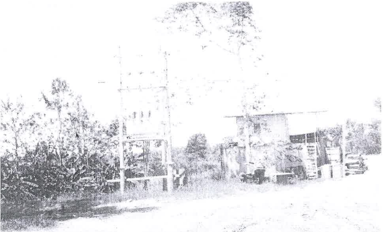
The step up transformer for the hydro electricity power that run the stone quarry project area
