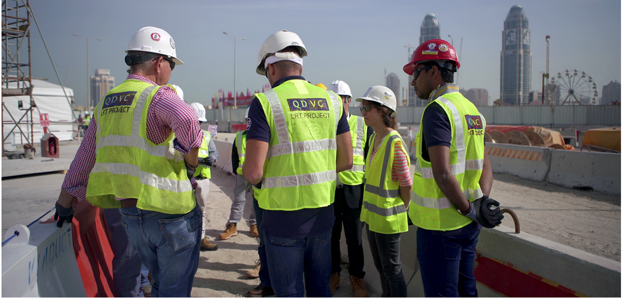
Site visit of the QDVC Underground Pearl Station of the Lusail Light Railway Transit System Project site.
