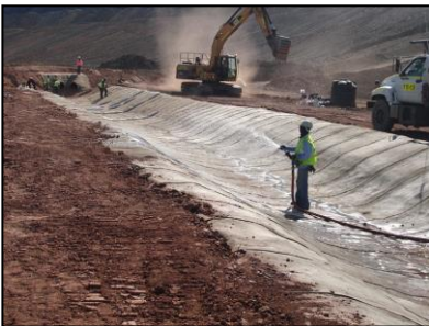
Lining installed.
