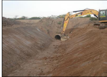
Upgrading the channel to install the lining.
